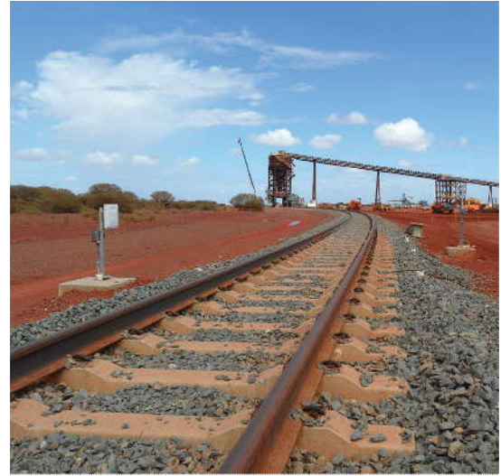
Inbound Train Identification point for TLI system at Christmas Creek.
