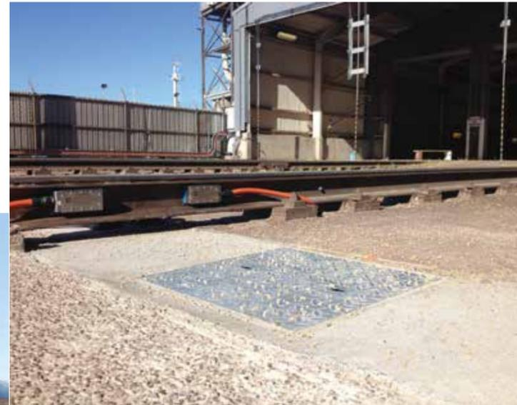
The heart of the TrackWeigh system, Meridian's patented bolt on load cell, at the Carrington terminal in Newcastle.
